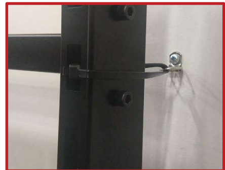
Figure 6: Rack secured to wall
